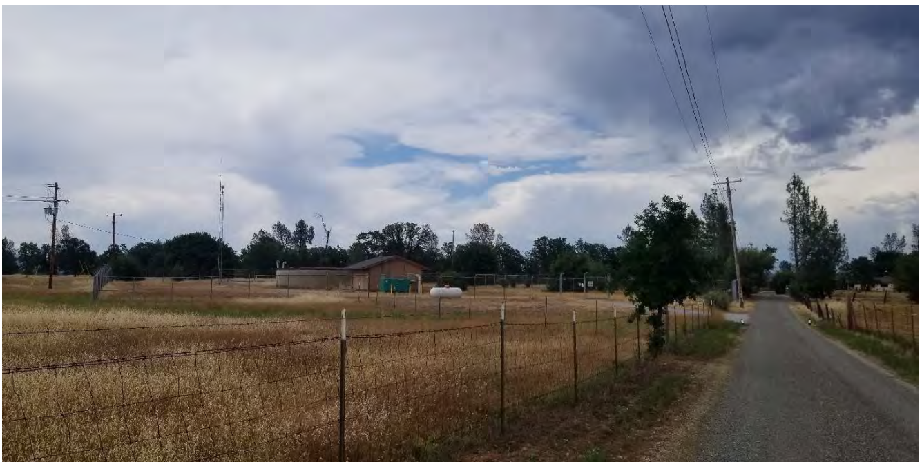
Photo 1. Regulating Station and Tank; facing east from Hidden Acres Road. June 6, 2023
